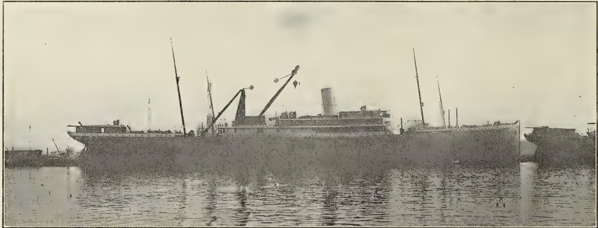
THE ANCONA ALONGSIDE CRANES FOR INSTALLATION OF BOILERS AND FUNNEL.
